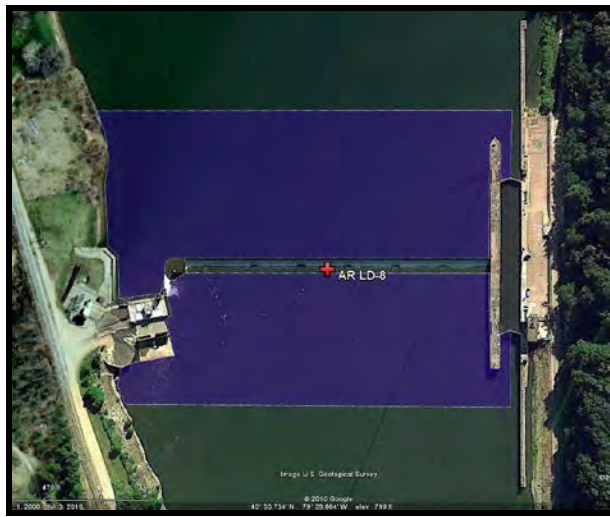
AR Lock & Dam # 8 Survey Coverage Area
