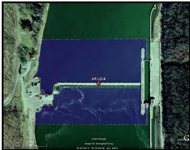
AR Lock & Dam # 9 Survey Coverage Area
