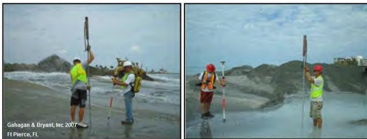
Figure 11-14. Setting a metal grade stake with driving hammer during active beach fill construction. Pre-drilling the stake hole with a portable auger makes for easier driving. RTK stake out observations are used to determine grade levels relative to the template along the profile range. Ft. Pierce Beach Renourishment Project. (Jacksonville District)
